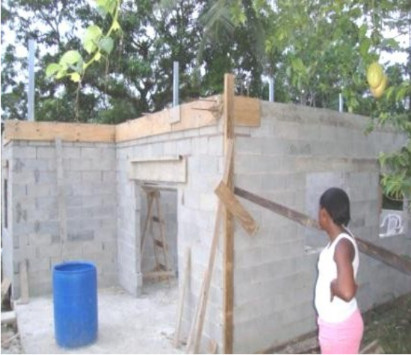
Cathy inspects house under construction
